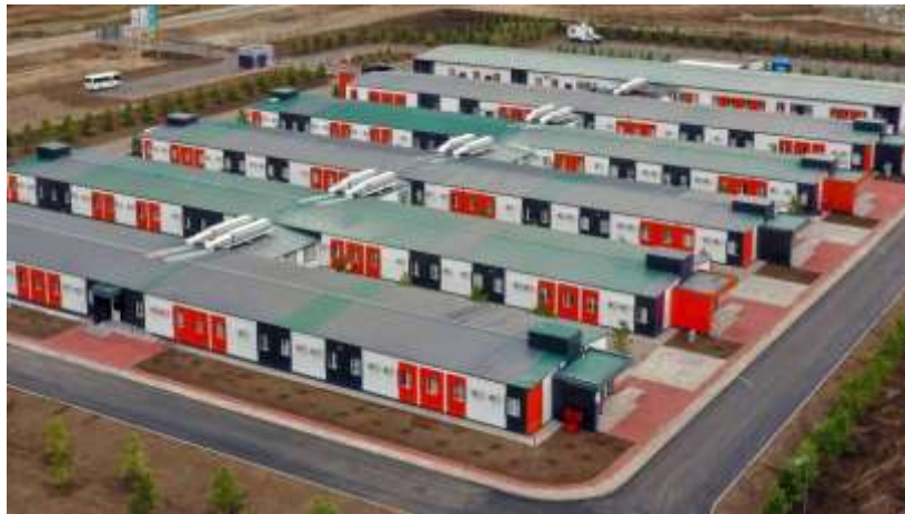
The hospital in Nur-Sultan, assembled out of modular blocks using the technologies for constructing prefabricated buildings, is designed for 200 beds. [Twitter]
